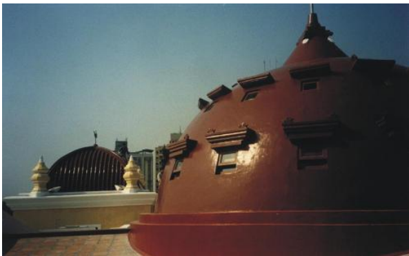
Figure 4. Details of the Saint Joseph's Church dome. Source: author.
